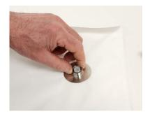
i) Engage and hand-tighten the connector without forcing it
